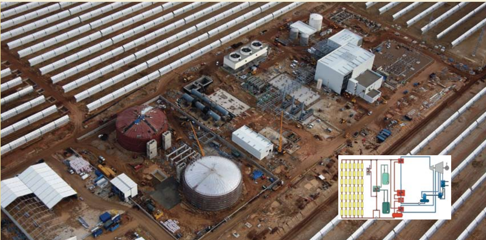
Solar-salt plant, Spain
