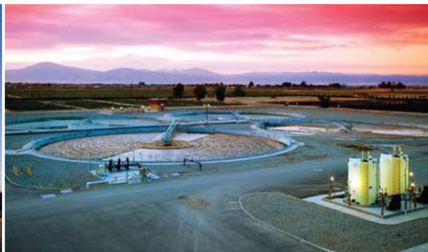
Bakersfield Wastewater Treatment Plant 3 – Bakersfield, CA
